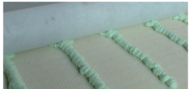
A bonded membrane incorporating HardRock Multi-Fix (DD)
