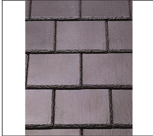
1.2 The slates are available in the natural colours of grey, green and heather. Slight colour variations may exist between batches; therefore, slates should be randomised on site to achieve a consistent appearance when installed.
